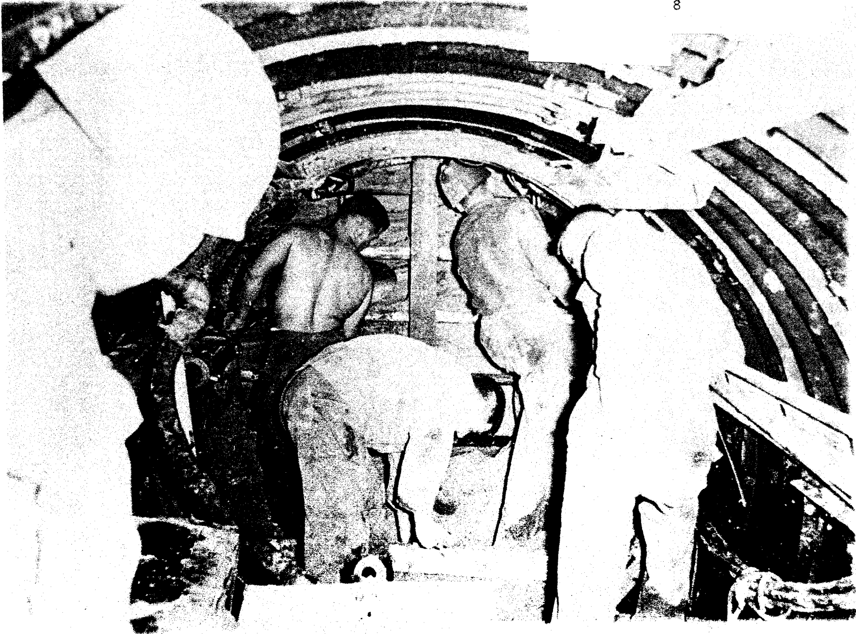
Figure 8 - Excavating Using the Blinds
