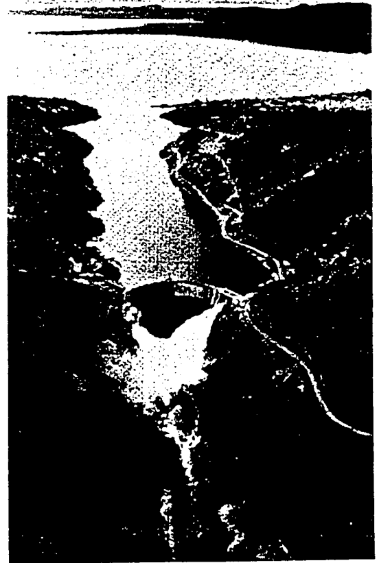
Delcommune: one of four major hydroelectric powerplant complexes producing electricity for the Copperbelt
