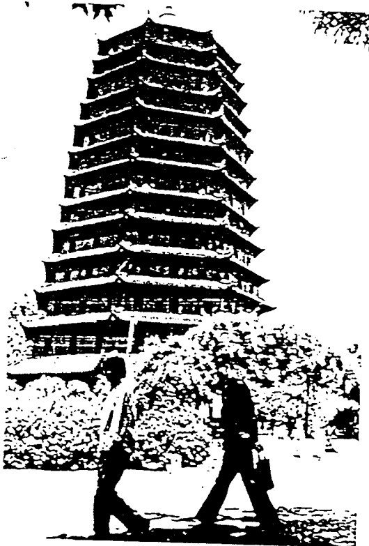
Figure 12. Liu-ho T'a (Pagoda of the Six Harmonies). The pagoda, one of the largest in China, is on Yueh-lun Shan (Moon Wheel Hill) overlooking the Ch'ien-t'ang Chiang, south of Hang-chou. In China, the Six Harmonies are the four compass points and up and down. The present 200-foot structure is built of brick and faced with wood.
