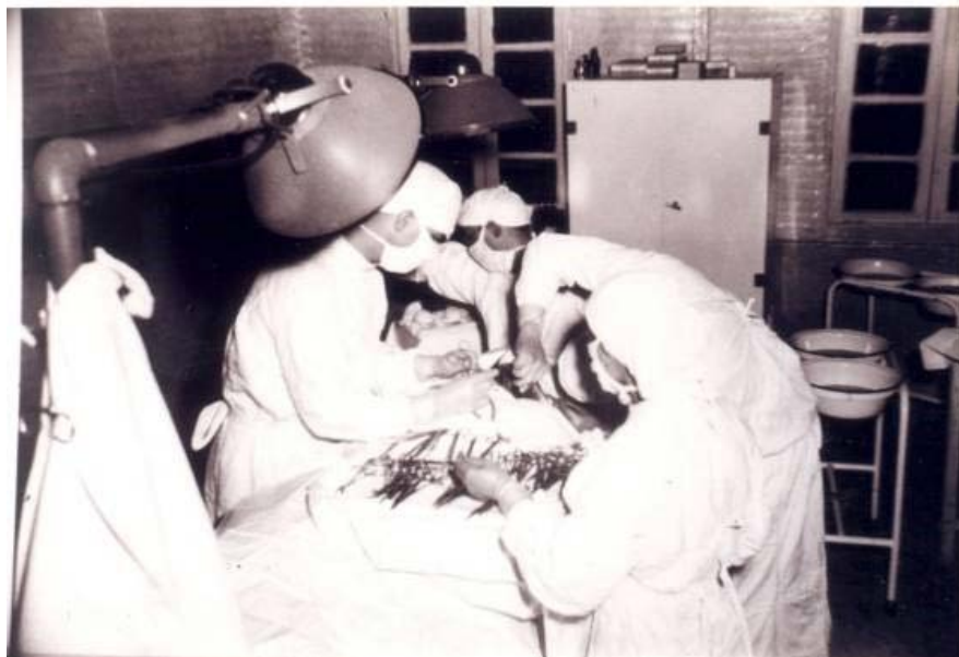
Nazira hospital operating room. Photo: Personal collection of Troy Saquety.
