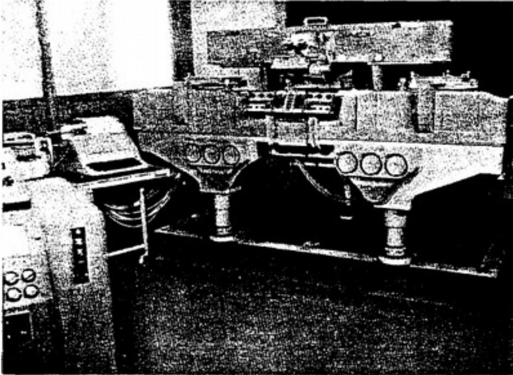
Figure 3. Nistri Stereocomparator TA-3.
